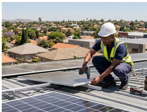
Solar and backup power equipment
