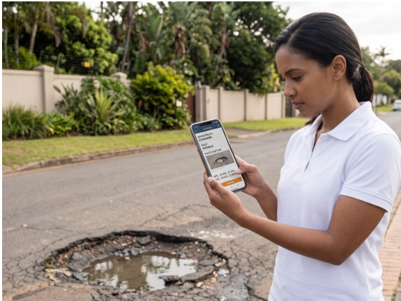
Municipal fault reporting in the field
